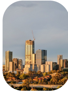
Heat Control Parramatta, Australia
